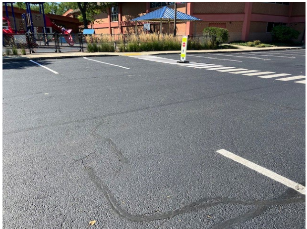
Crews seal coated and crack filled the parking lot at the Community Recreation Center.
