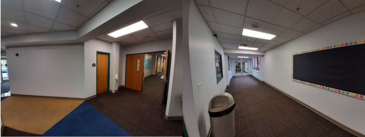
Painted the hallways within the Early Childhood wing at Community Recreation Center.
