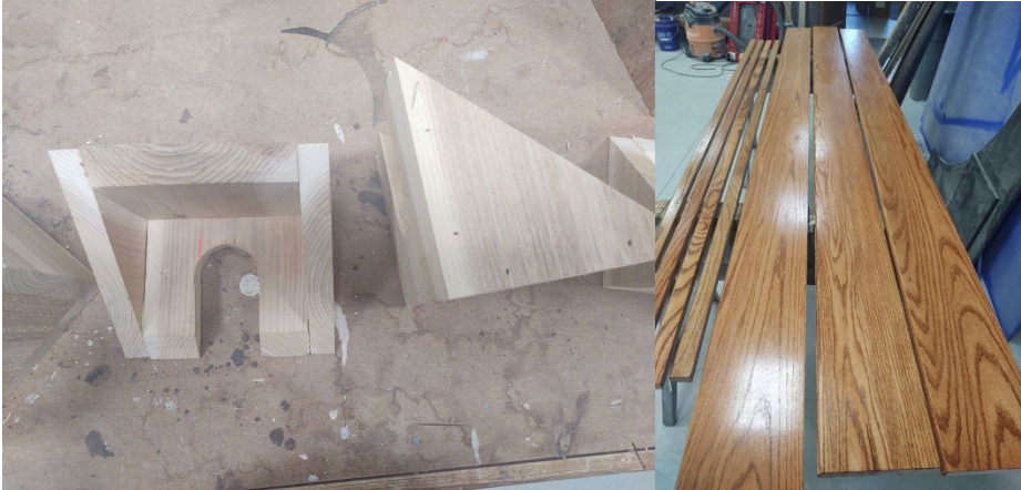
Built custom wire covers for the golf restaurant pendant light and installed the floor trim.
