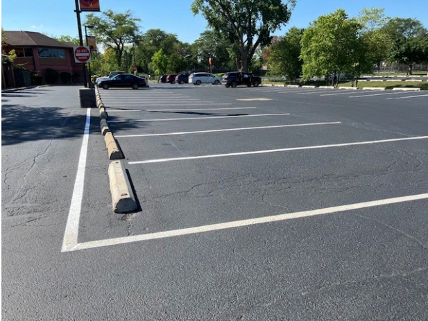
Crews seal coated and crack filled the parking lot at the Community Recreation Center.
