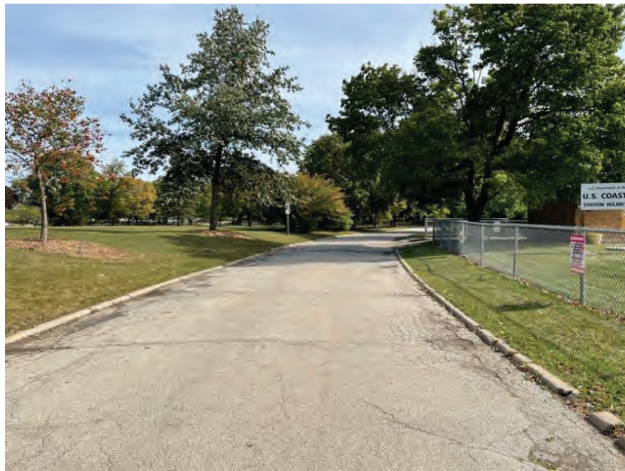
EXISTING HARBOR DRIVE CONDITION
