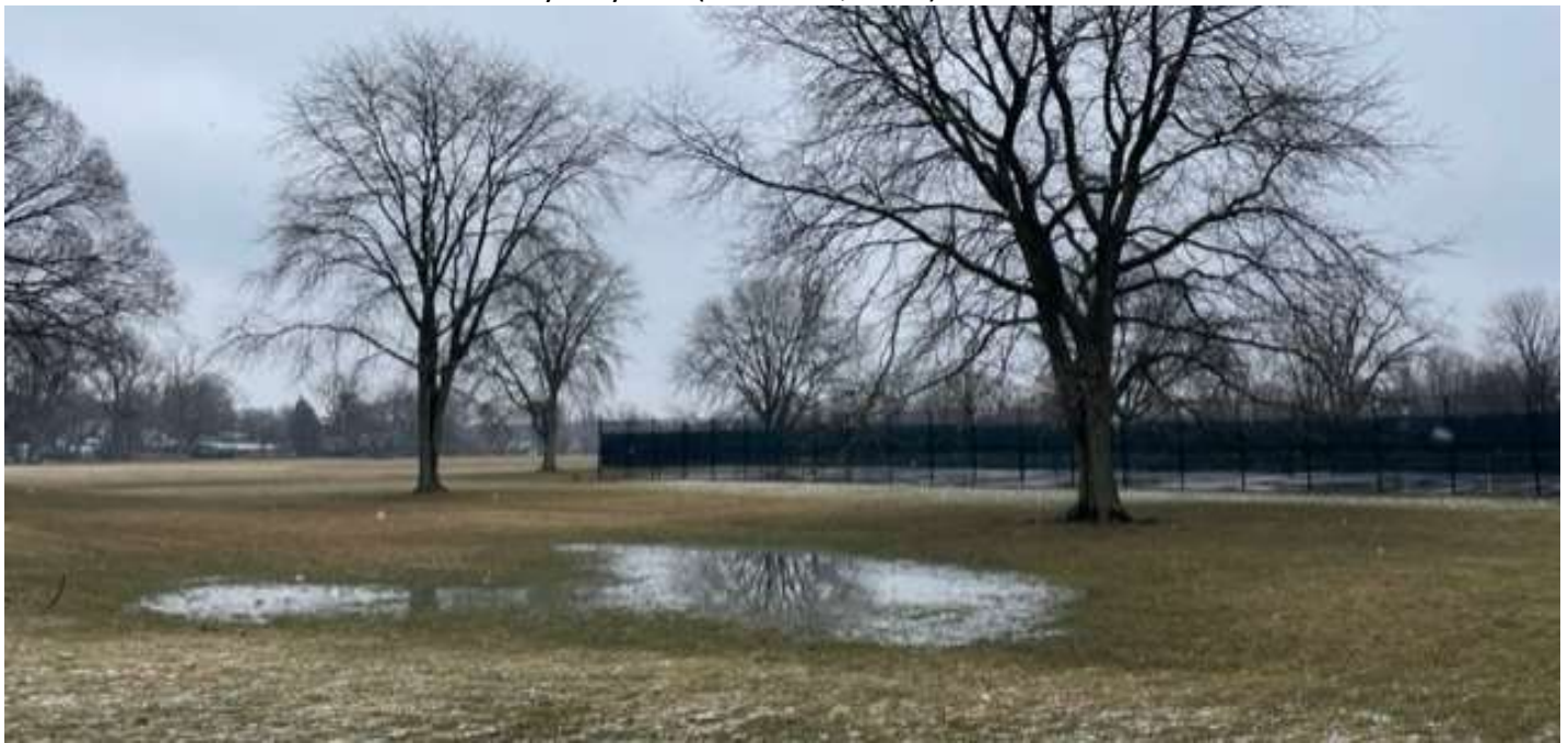
Photo E: stormwater in The Community Playfield (March 12, 2023)
