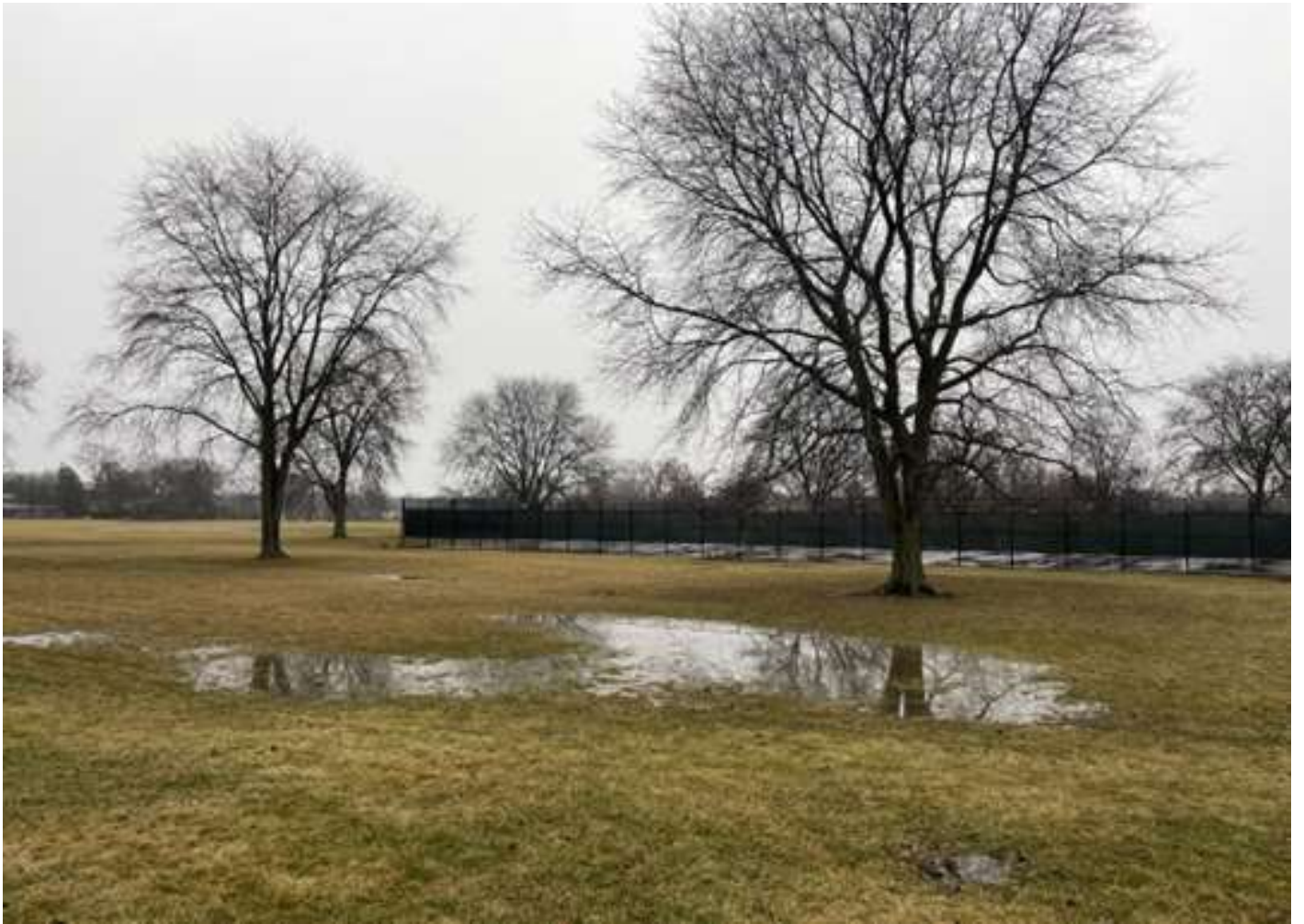
Photo A: stormwater in The Community Playfield (February 9, 2023)
