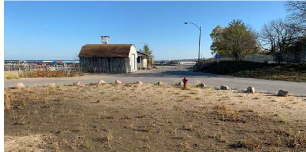
Parking lot bioswales have lost a significant amount of vegetation due to flood and drought conditions. Sand, soil, and mulch have washed and eroded away.
