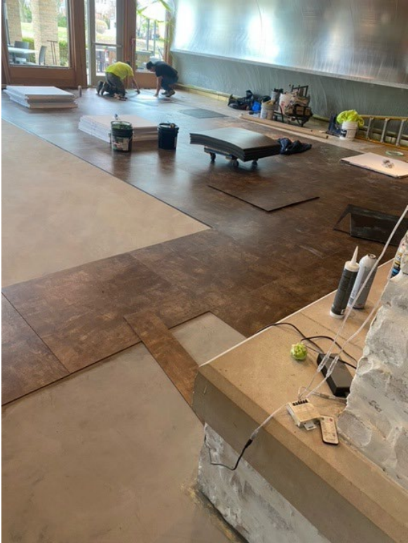
Golf-Installed flooring in the clubhouse.
