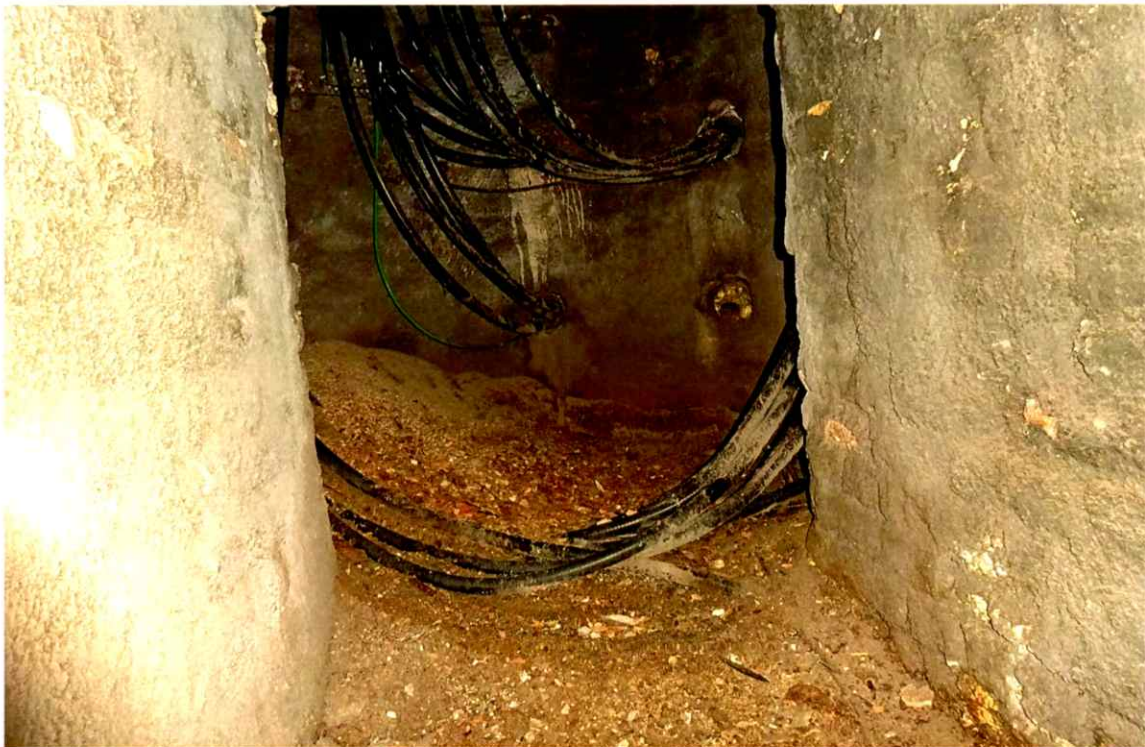
Photo 82. Good interior condition of the guniting tunnel inside the cleanout door.
