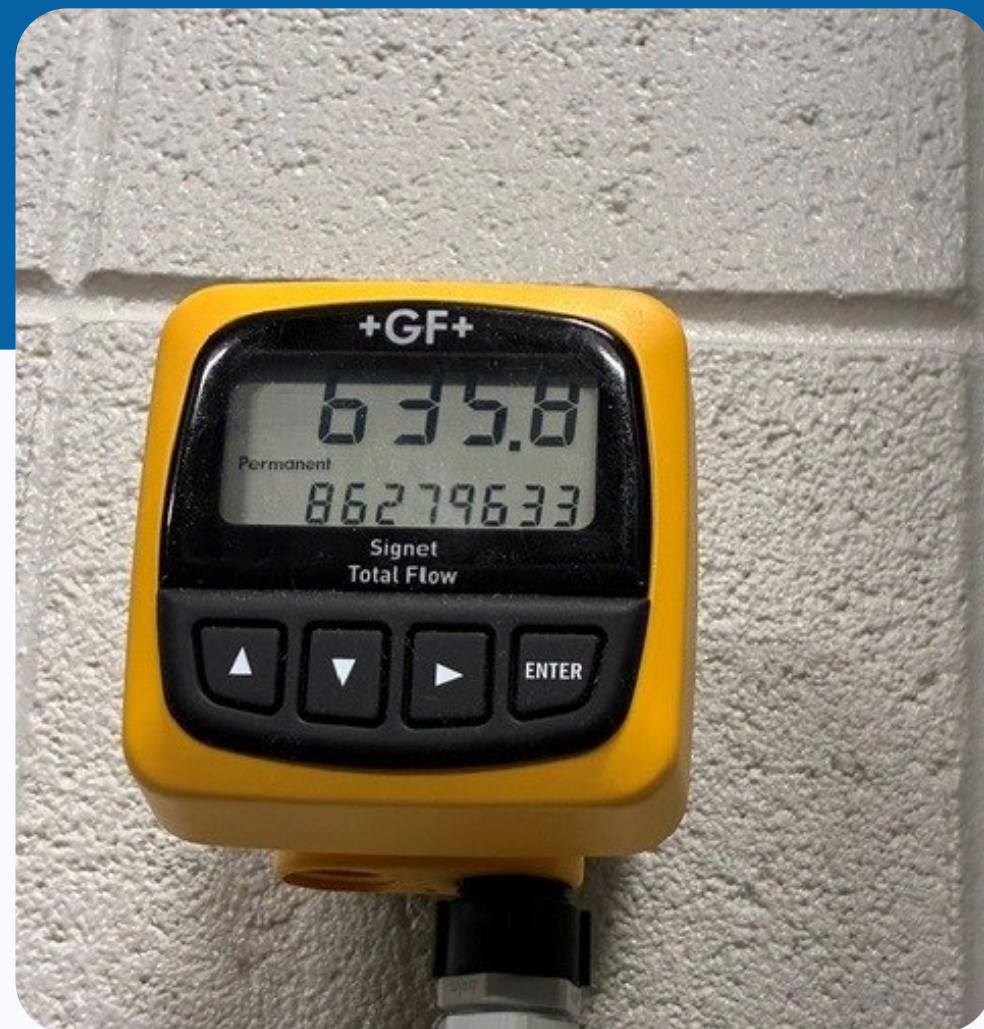
New flow meters installed
